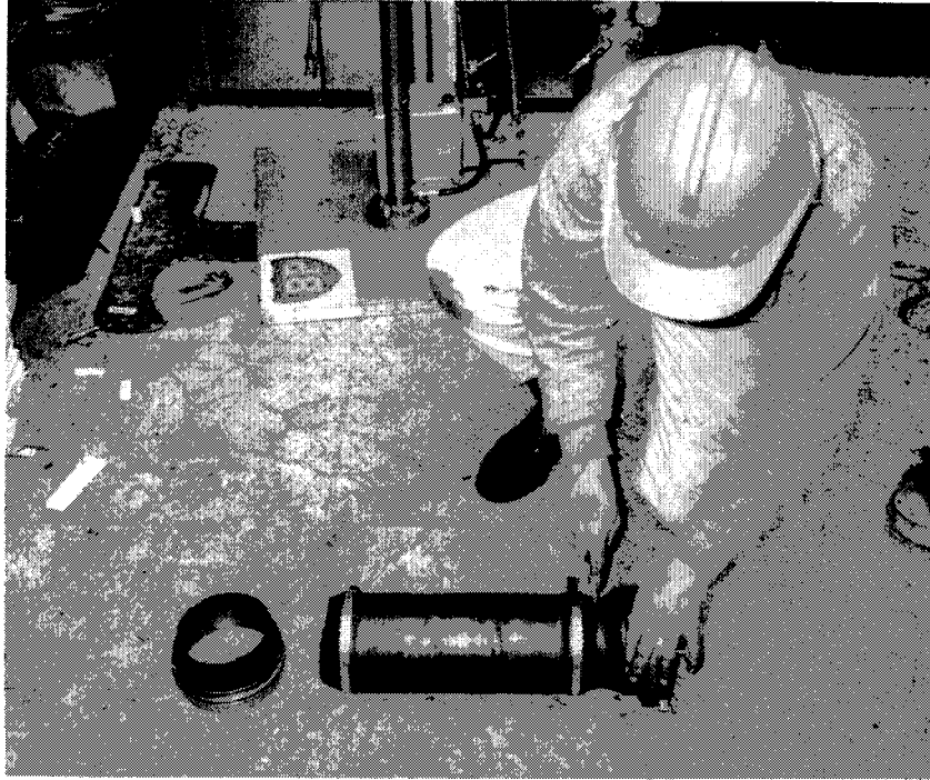
FIGURE 3 Trimming SST sleeves to length
