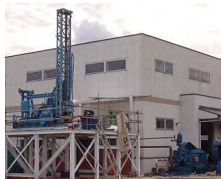
Figure 4: Drilling system for field tests
